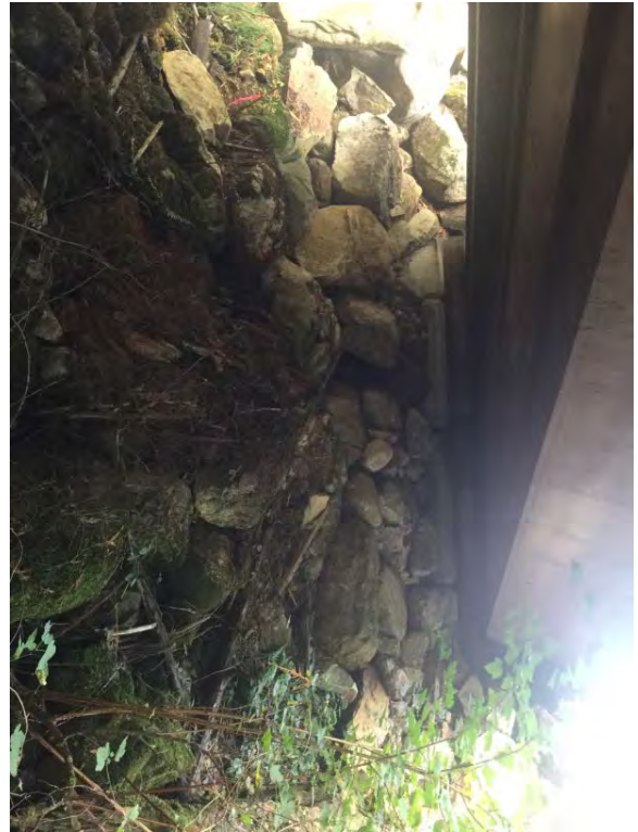
Right Bank Abutment when facing downstream
